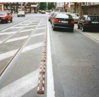
Hol - Separator 70'-120' is an element of road safety used for marking bicycle lanes, separating tramway rail tracks from vehicle lanes, designation of parking spaces, separation of bus bays, etc.
